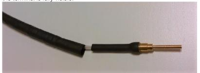
Place the tube so that it partially covers the small rubber section of the existing fiber terminal.
